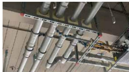
Short stubs to and from radiators, connected to relatively long straight runs should also be avoided. This can usually be achieved by introducing an expansion loop, thereby increasing the length of pipework fixed between the flow/return legs and the radiator connection. However, expansion accommodation techniques such as the use of loops and horseshoes may not be sufficient to accommodate large expansions and in such cases the use of the bellow type couplers may be necessary.
