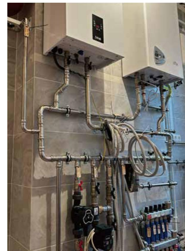
ConfitPRESS with black EPDM sealing rings are suitable for use cooling and refrigeration circuits in closed and open versions with operating temperatures between -20 / +120 °Centigrade.
